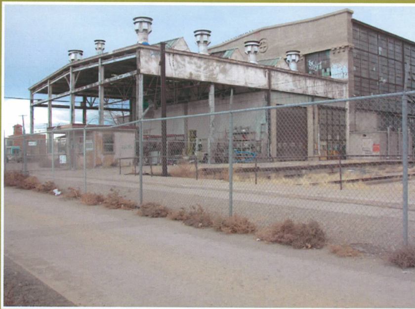
Firing Shed at west end of Boiler Shop with two bays converted to paint booths
